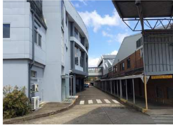
Figure 4. Existing industrial building
