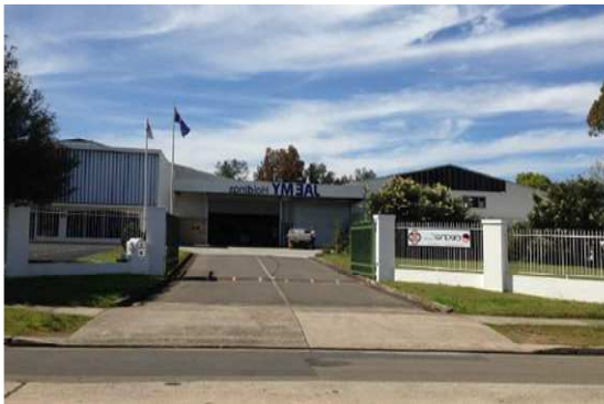
Figure 7. Existing building at 8 Wharf Road
