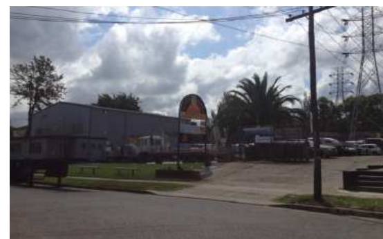
Figure 10. Industrial buildings on Hope Street
