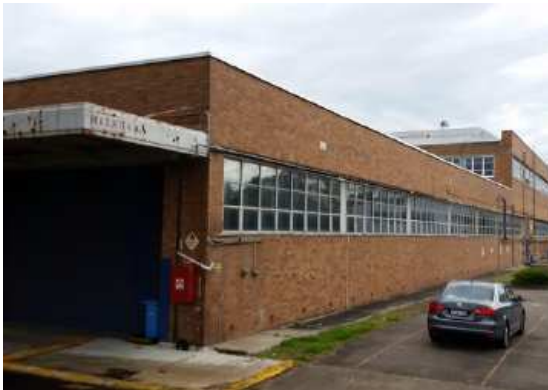
Figure 5. Existing industrial building
