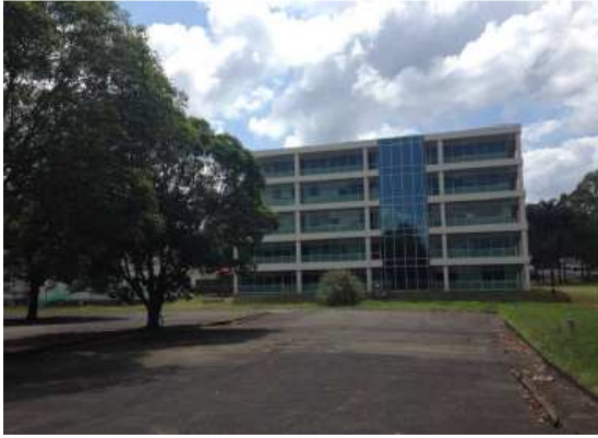
Figure 3. Existing industrial building
